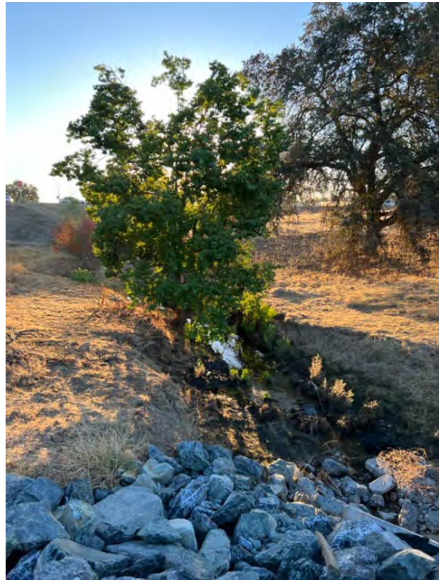
Photo #2, Tree #2359 on the right and #100 in the drainage channel on the left.
